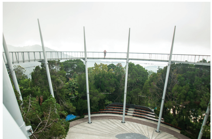
At the skywalk bridge at Penang Hill
